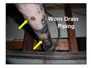
The underground waste piping that runs from the building to the main sewer may be older or original. Waste piping of this age is often worn or damaged in the underground portions. Old sewer piping is often blocked or damaged by roots and other obstructions. We recommend the sewer laterals be examined for defects by a qualified plumber using special video equipment designed for this purpose.
